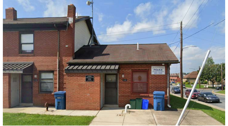
2. Bethlehem Police Department Northeast Sub Station
