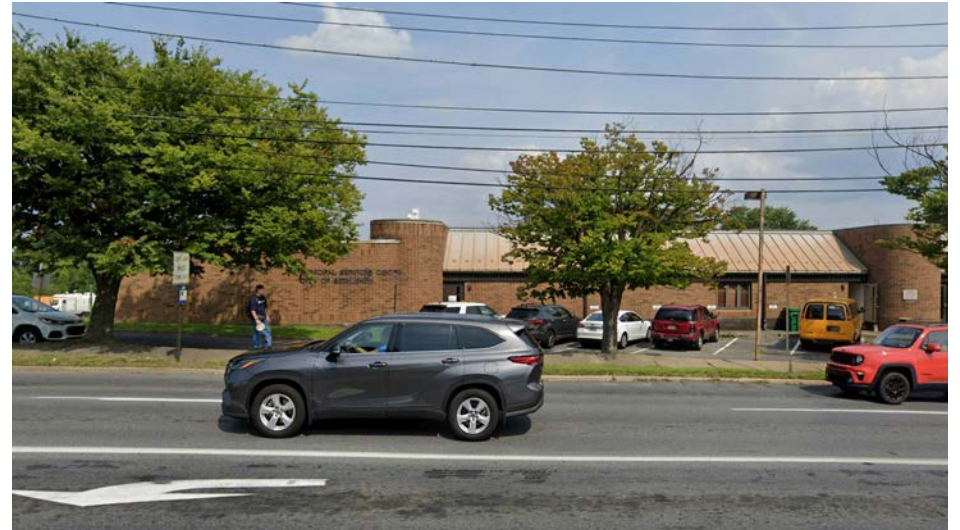
4. City of Bethlehem Municipal Services Center
