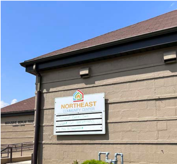
8. Northeast Community Center
