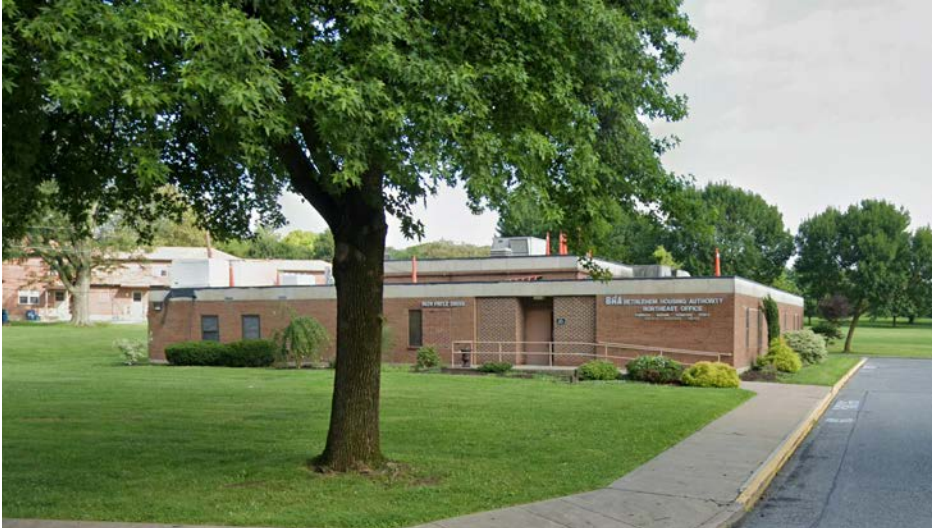
1. Bethlehem Housing Authority: Northeast Office
