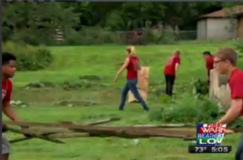
Project 1013 cleaning up
